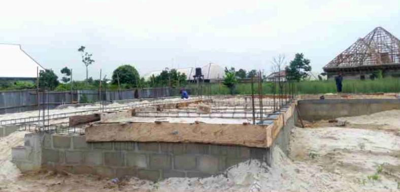
Ongoing construction of Okerewa Community Health Centre at DPC stage.
